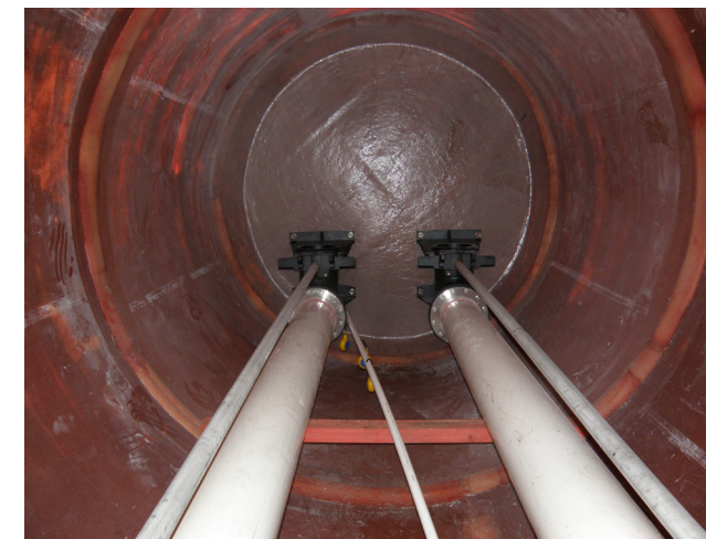
Fibreglass pump stations with dual guide rail fitout
