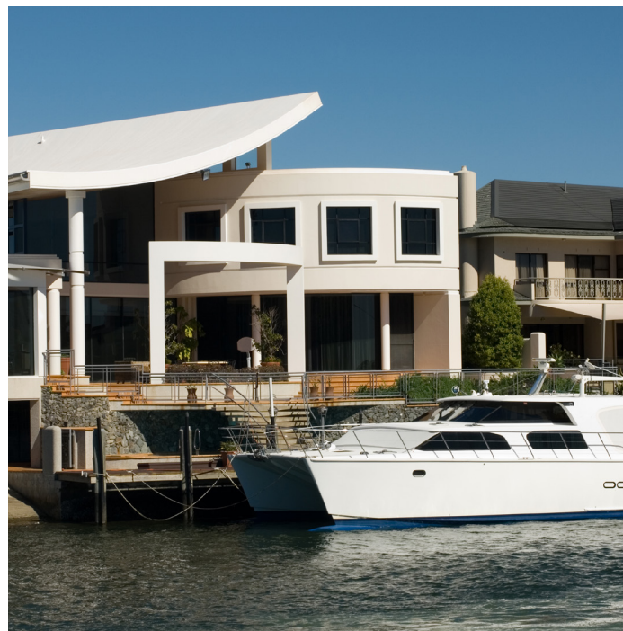
HOUSES WITHOUT FALL TO SEWER MAIN
