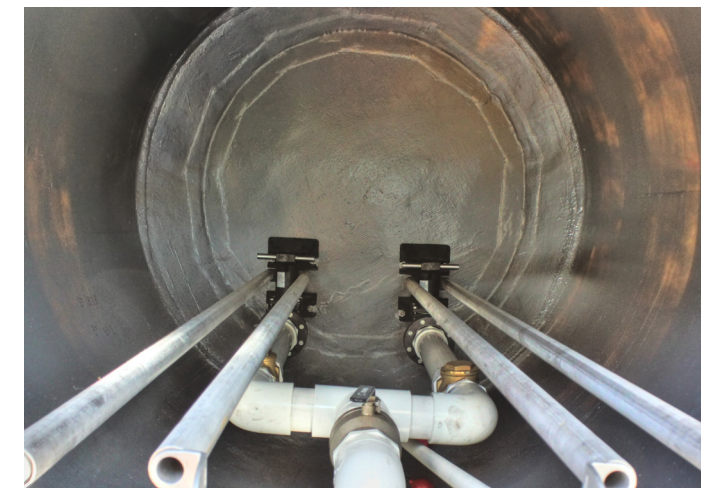
Fibreglass pump stations with dual guide rail fitout
